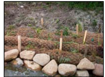
Biologs installed. Photo courtesy of JF New.
