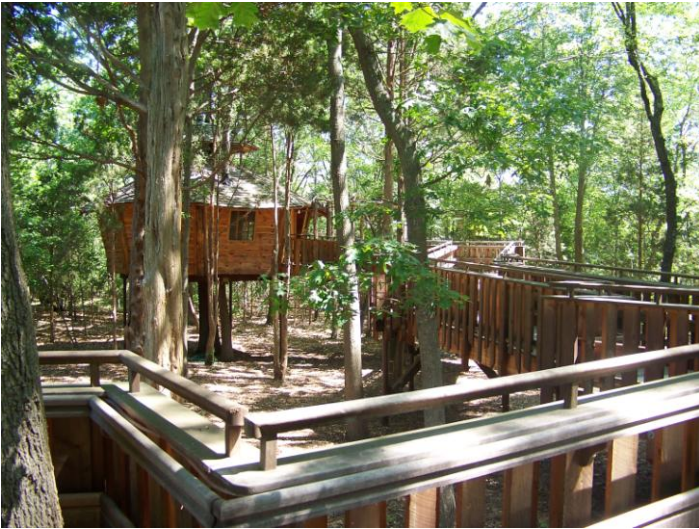
Tree House Construction
